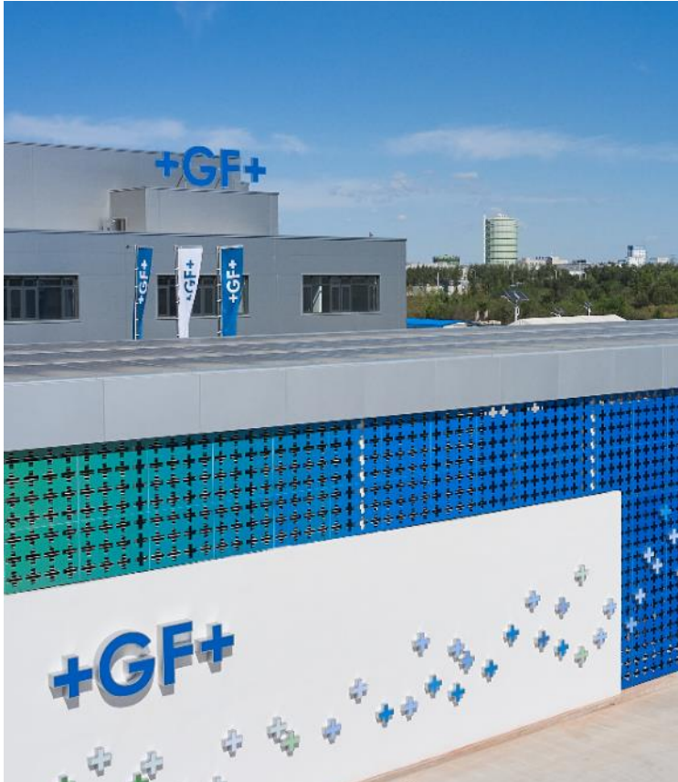
New plant in Shenyang (China) in full operation
